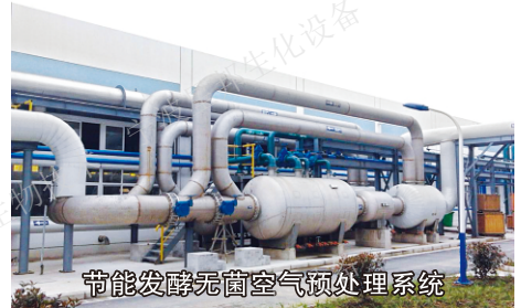
System of Fermentation Sterile Air Pretreatment (SAS)
